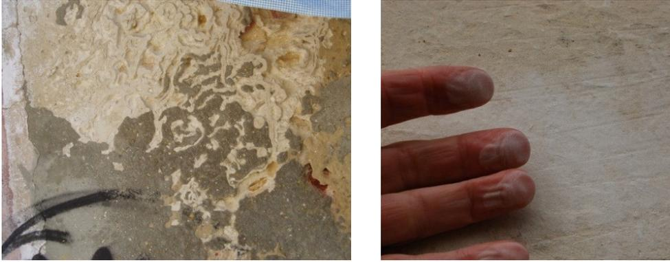
Fig. 3 Powdering (resulting in alveolisation) and chalking of plasters
