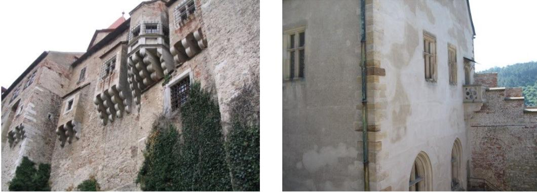
Fig. 1 Example of a situation in practice: disintegrated and partly detached aerial lime render before consolidating treatment (l), hydraulic lime render after consolidation and repairing (r)
