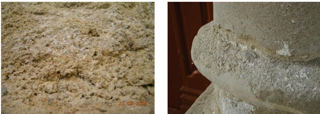
Fig. 2 Crumbling and sanding of plasters
