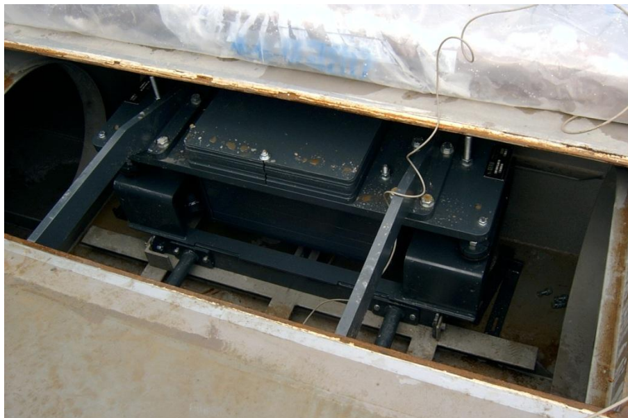
Figure 18: The installed absorber (TMD) inside of the box girder.
