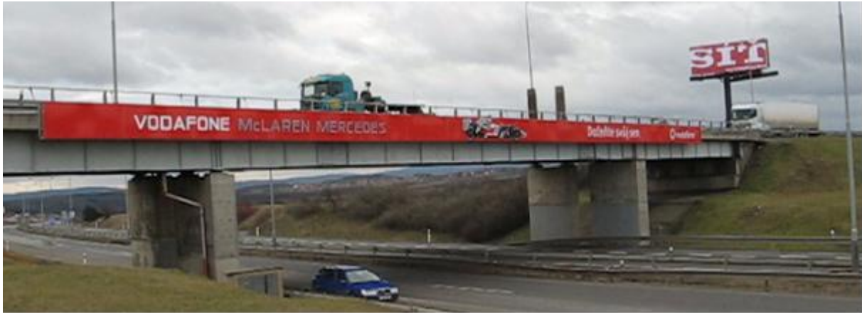
Figure 26: Two heavy trucks, which caused dynamic response of the investigated bridge (Fig. 27).
