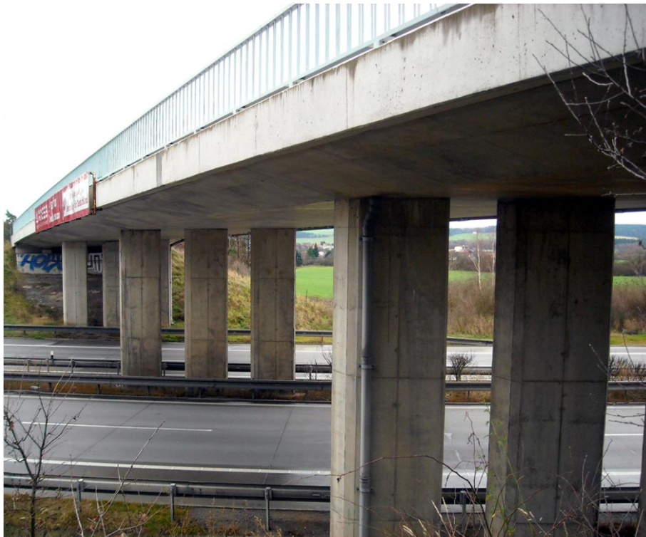
Figure 8: The view on the prestressed concrete slab bridge near the village Heřmanova Huť.
