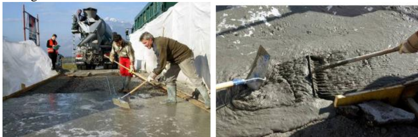
Figure 9 : UHPFRC for rehabilitation- easy application with usual tools
