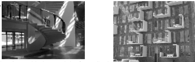
Figure 8: Spiral stairs and balcony slabs from CRC
