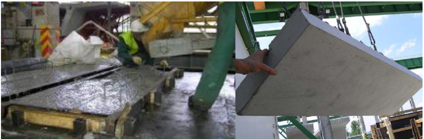
Figure 19 Filling of the forms
