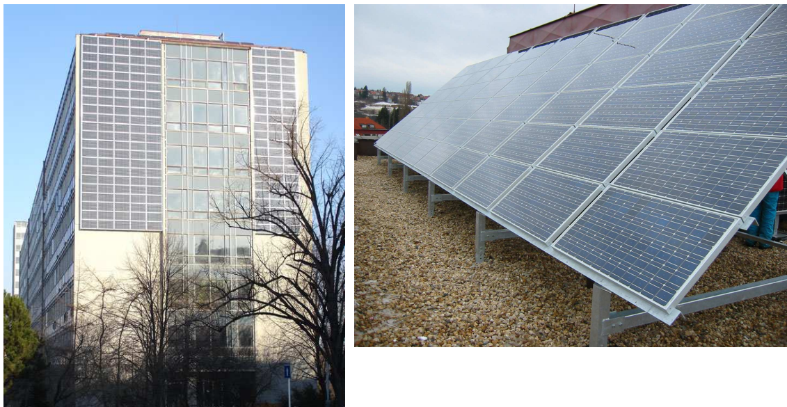
Fig.24 Ventilated PV facade at FCE CTU and a part of roof installation.
