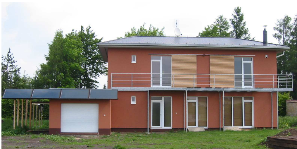
Fig. 20 House F (design J.Tywoniak et al.) with expected specific heat use for space heating by 30 \text{ kWh}/(\text{m}^2\text{a}) . The windows area: SW 30 %, SE 12 %, NE 6 % of particular façade.
