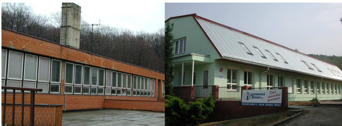
Fig.12 Kindergarten in Ostrava-Proskovice before and after refurbishment (pitched roof is covered by roof integrated solar collector- 120 m 2 )
