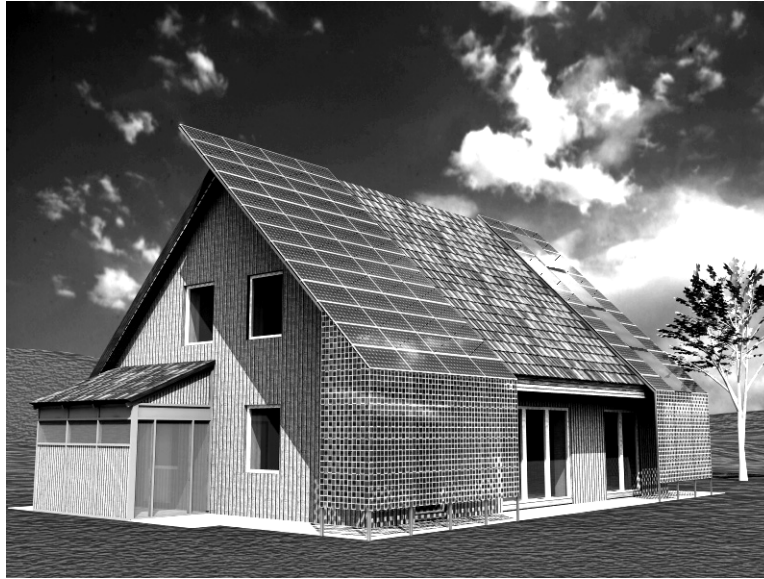
Fig.16 Study of solar-optimized solution for a passive house at close-to-zero energy level (developed from a real design of passive house [12]). The PV system covers the entrance area of the building and also the adjacent roof (independent structure guarantees good ventilation of solar panels fixed). Other smaller parts of the PV systems, i.e., those that are semi-transparent, are situated in a vertical position in front of the facade. Solar thermal system is integrated in the roof together with PV panels in strips near the gable wall.
