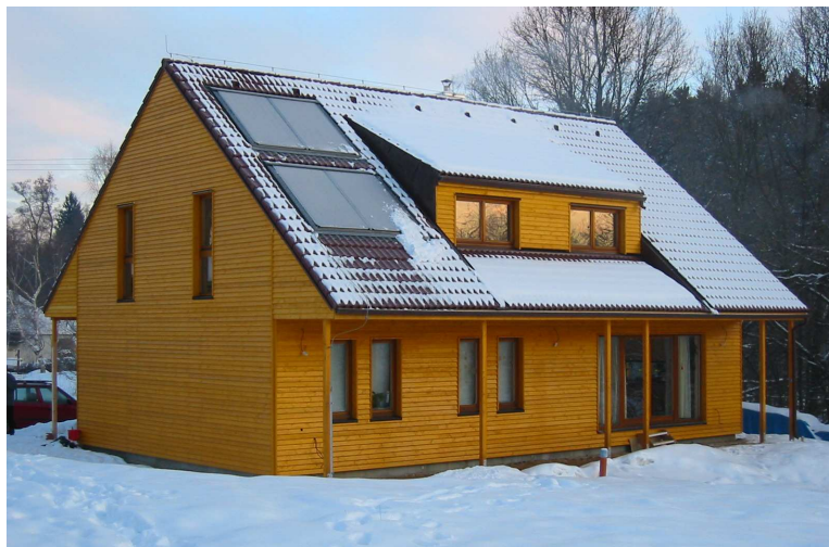
Fig. 17 House W (design M.Šenberger, J.Tywoniak, et al.) built 2003. Low-energy house ( 44 \text{ kWh}/(\text{m}^2\text{a}) ) using passive house components: mechanical ventilation with efficient heat recovery, earth heat exchanger 21 m, 1 \text{ m}^3 water accumulator in service room, integrated solar system (net area 8,1 \text{ m}^2 ) + electric heating rods, additional local heat source in living space (wood).
