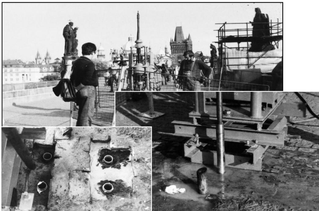
*Fig.19: Drilling of boreholes in Charles Bridge*
