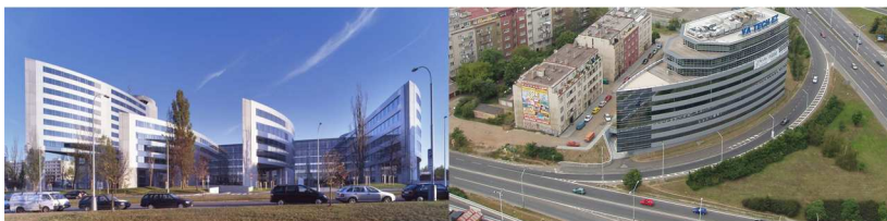
obr. 4 budovy Kavčí Hory Office Park a Polygon House
