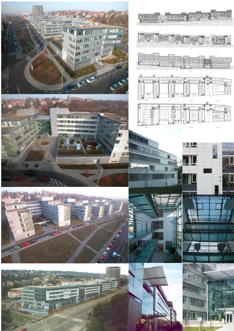
obr.23 Office Park Hadovka, Praha 6
