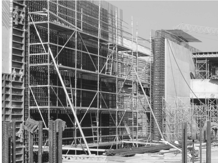
Figure 15: Investigated wall with formwork
