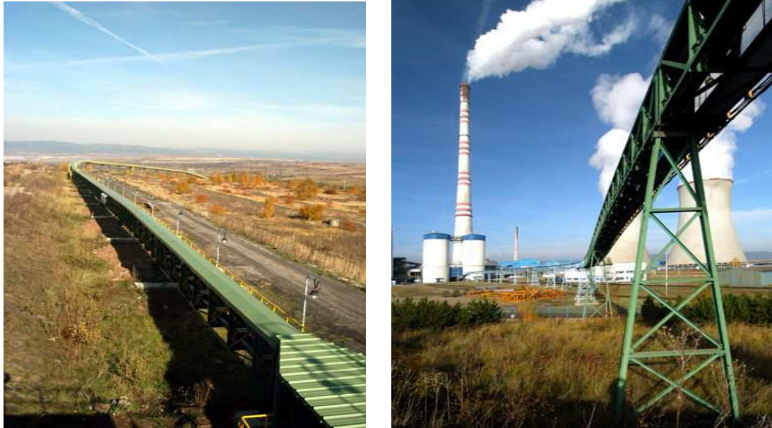
Figure 1. Slurry pipeline conveying ash and slag from the Tušimice II power plant to a disposal site (source: Hochtief web site).
