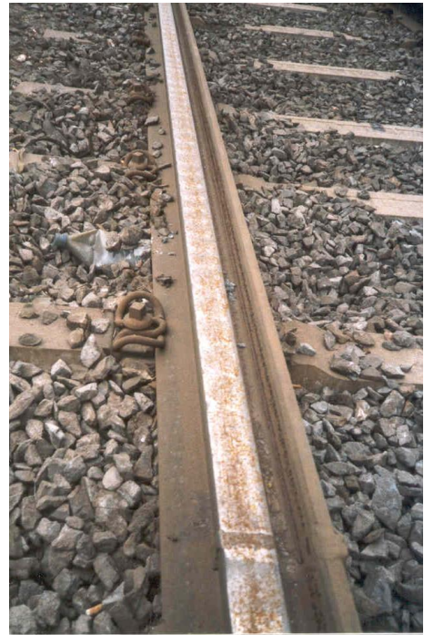
Fig. 5 Wavelets on the rail head surface and bad rail joint
