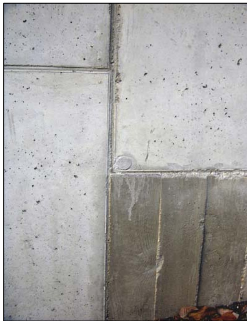
Fig. 1 Fair-face concrete surface
